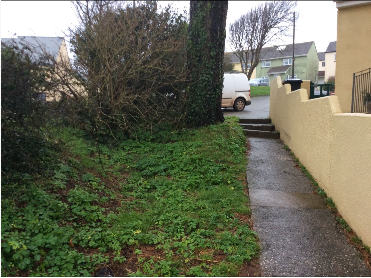
Figure 3: Point of origin from linear POS and condition of footway serving properties
